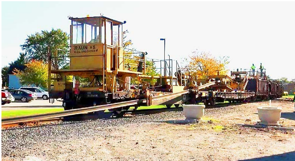
RAUN Rail Unloading Train with Rail Shute; USA
