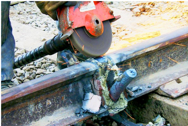
Finishing, Stripping and Grinding of AT Rail Weld
