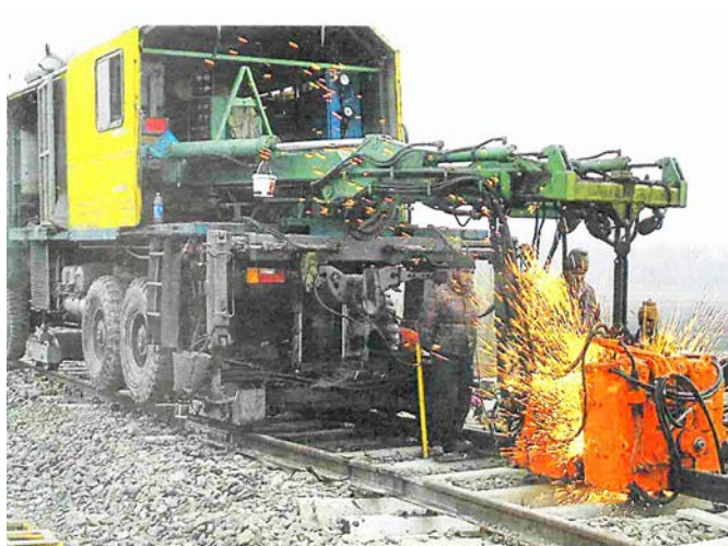
Mobile Flash-Butt Welding on Kashmir Valley Railway Line with Holland, USA, Flash-Butt Welding Unit; source: Northern Railway; India
