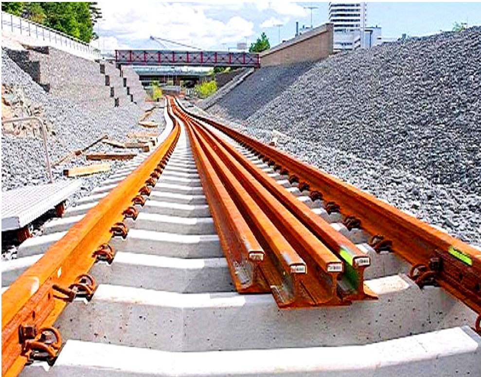
Laying new Track with Long Rolled Rails, LRR; pict.: Aloy Rumania
