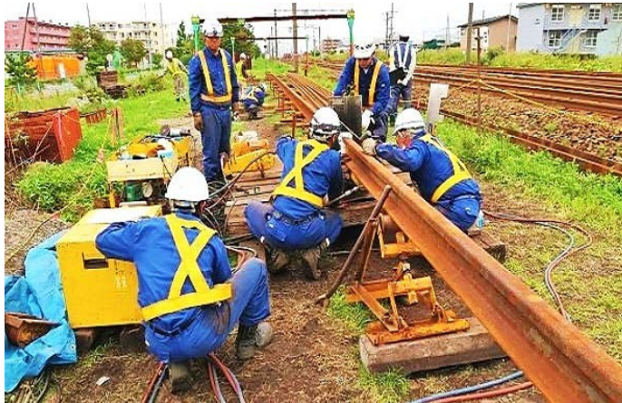
Gas Pressure Rail Welding at Site
