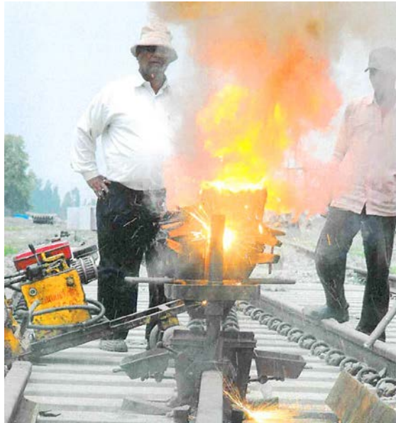
AT Welding on Kashmir Valley Railway Line; source: Northern Railway; India
