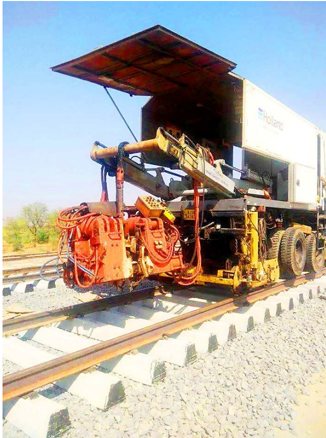
Mobile Flash-Butt Welding on Dedicated Freight Corridor with Holland RRV Mobile Flash Butt Welding Machine; Image: DFCCIL
