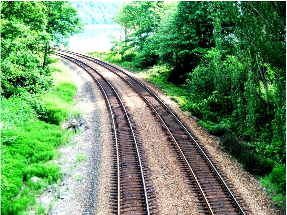
Continuous Welded Rail Track, CWR, with Long Rolled Rails, LRR; USA
