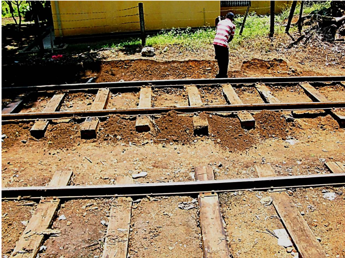
Fig. 26: Srilankan "EARTH-WORKS" for "BALLAST-LESS" Rail-Track; Pict. by F. Wingle
