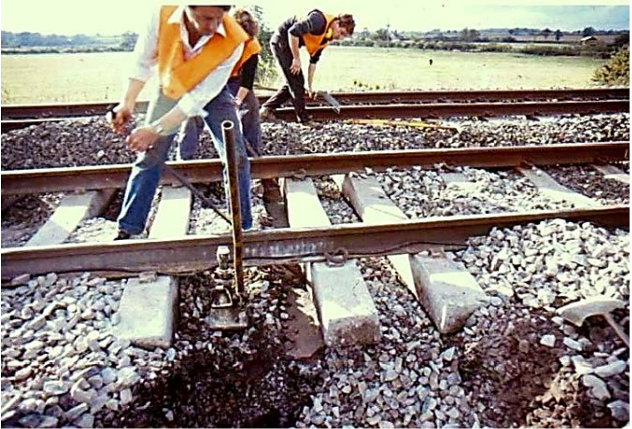
Fig. 20: Ballast Cleaning through manual “Deep-Screening”; Pict. by Andy Franklin, Carillion Rail, UK
