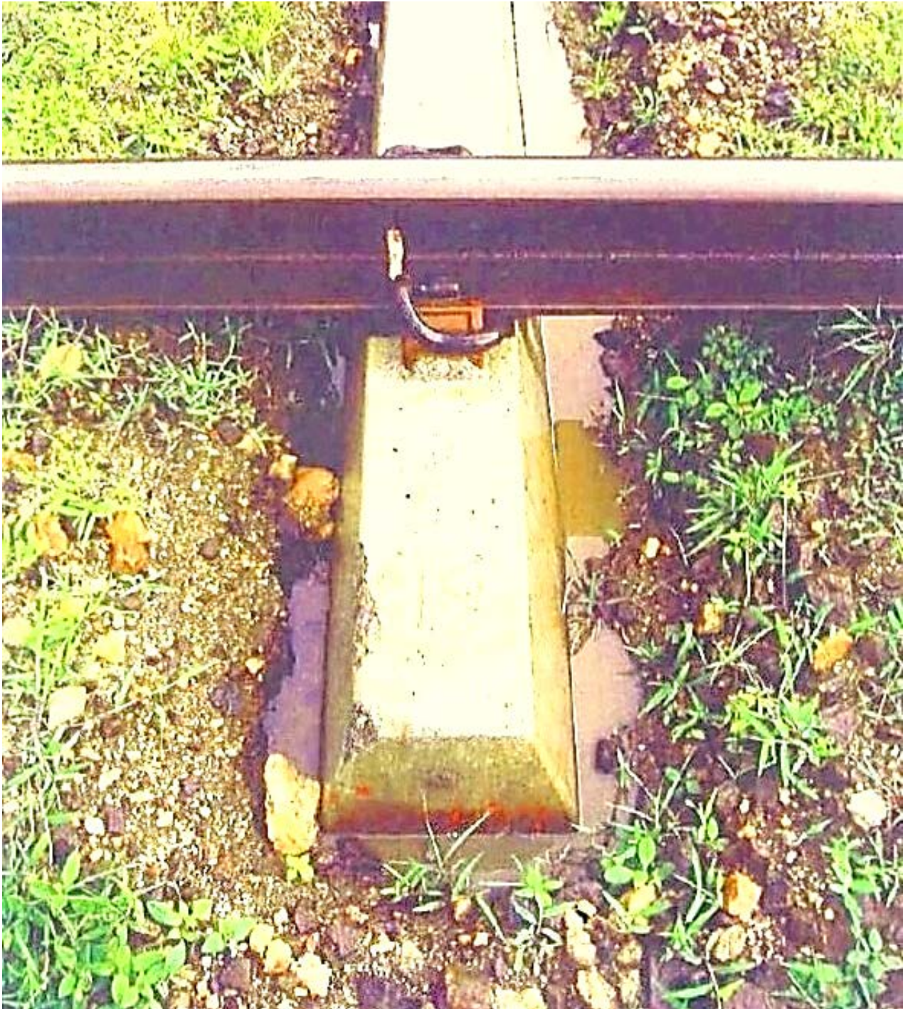
Fig. 5: Formation and Ballast Damage caused by Concrete Sleeper on poorly ballasted Track after Replacing Wooden Sleeper; UVA Railway; Pict. by F. Wingle
