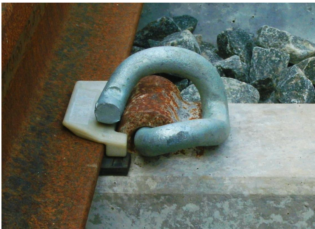
Indian Mark III ERC Clip inserted with the Leg in the Shoulder-Plate Housing the wrong Way on Indian Concrete Sleeper with Indian Shoulder Plate on a short temporarily laid provisional and warped Demonstration-Track with insufficient Sub-Ballast, Ballast-Cushion and Ballast-Shoulders between Matara and the Nilwala River Bridge for a political Track-Laying Ceremony on January 12 th 2018
