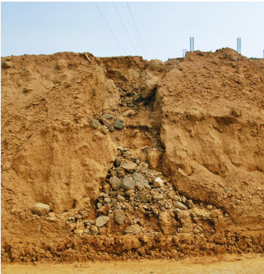
Heavy Slope Corrosion at Landfilling for Beliatta Railway Station
