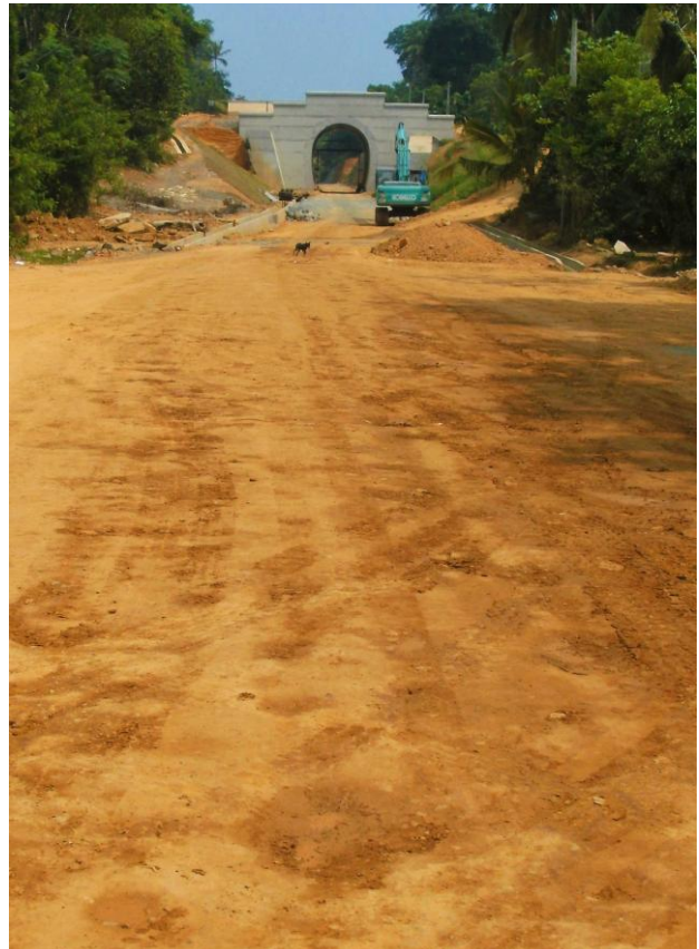
Earth- and Sub-Grade Works in Progress near new Wewurukannala Railway Station
