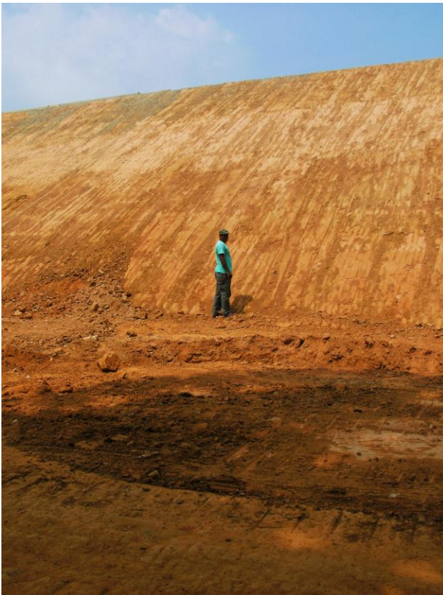
Unsettled fresh Embankment Filling between Wewurukannala and Beliatta
