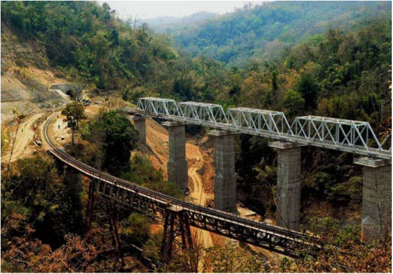
Meter to Broad-Gauge Conversion in the Cachar Hills on the Lumding-Silchar Route, Assam
