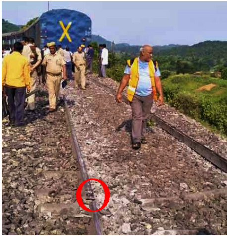
Rail-Fracture on a poor Quality Rail-Track in Need of “Fire-Brigade” Track Spot/Patch- Repair
