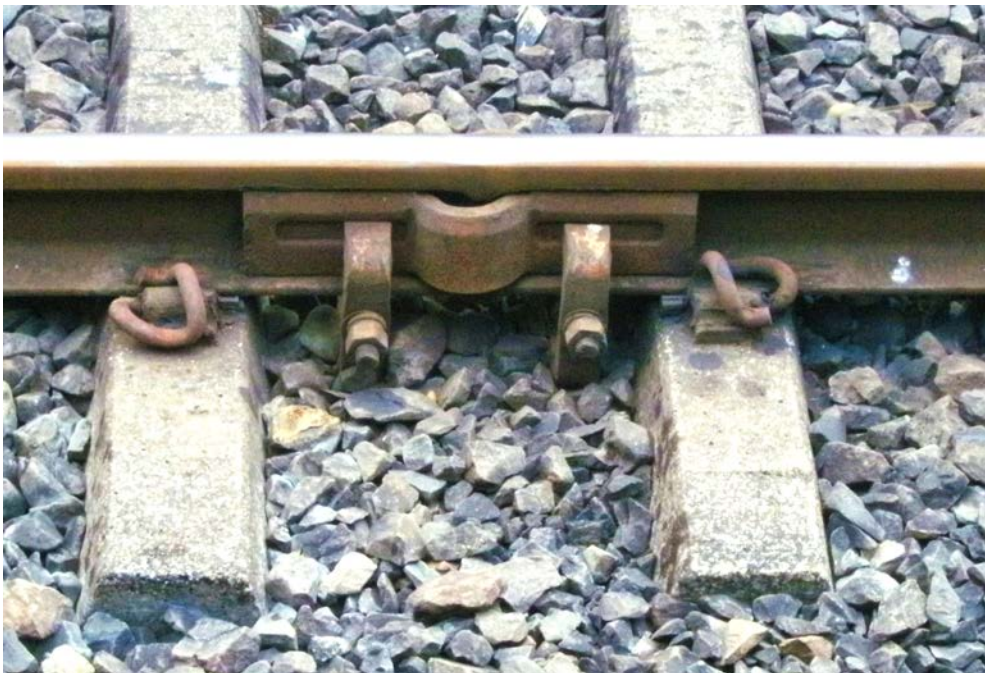
AT weld, bandaged with Joggle Fish-Plate, Konkan Railway, October 2017
