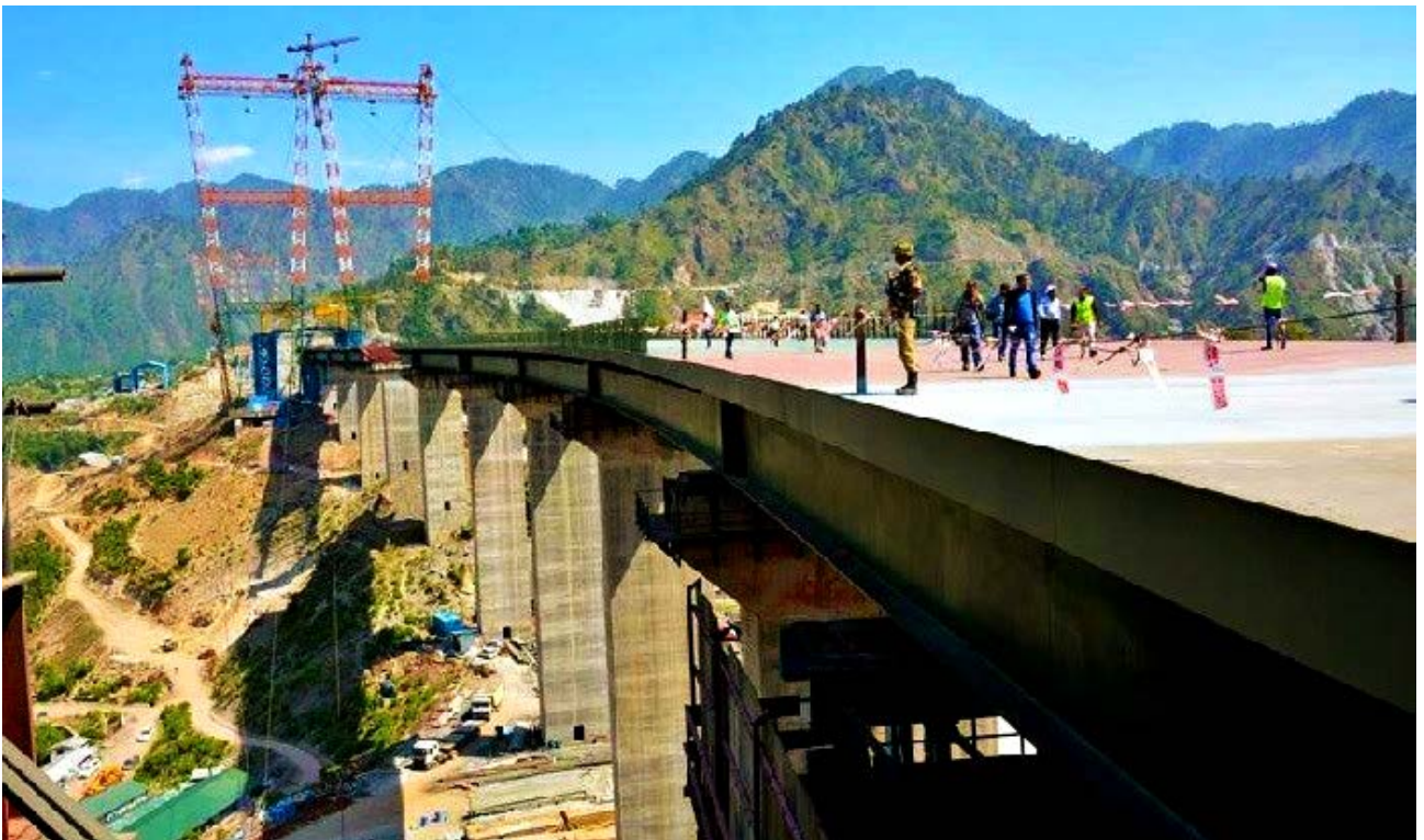
Chenab-River Bridge under Construction
