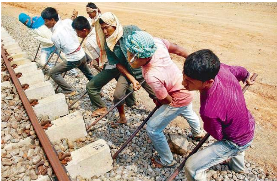
Outdated manual Labour Work for high Quality Tracks
