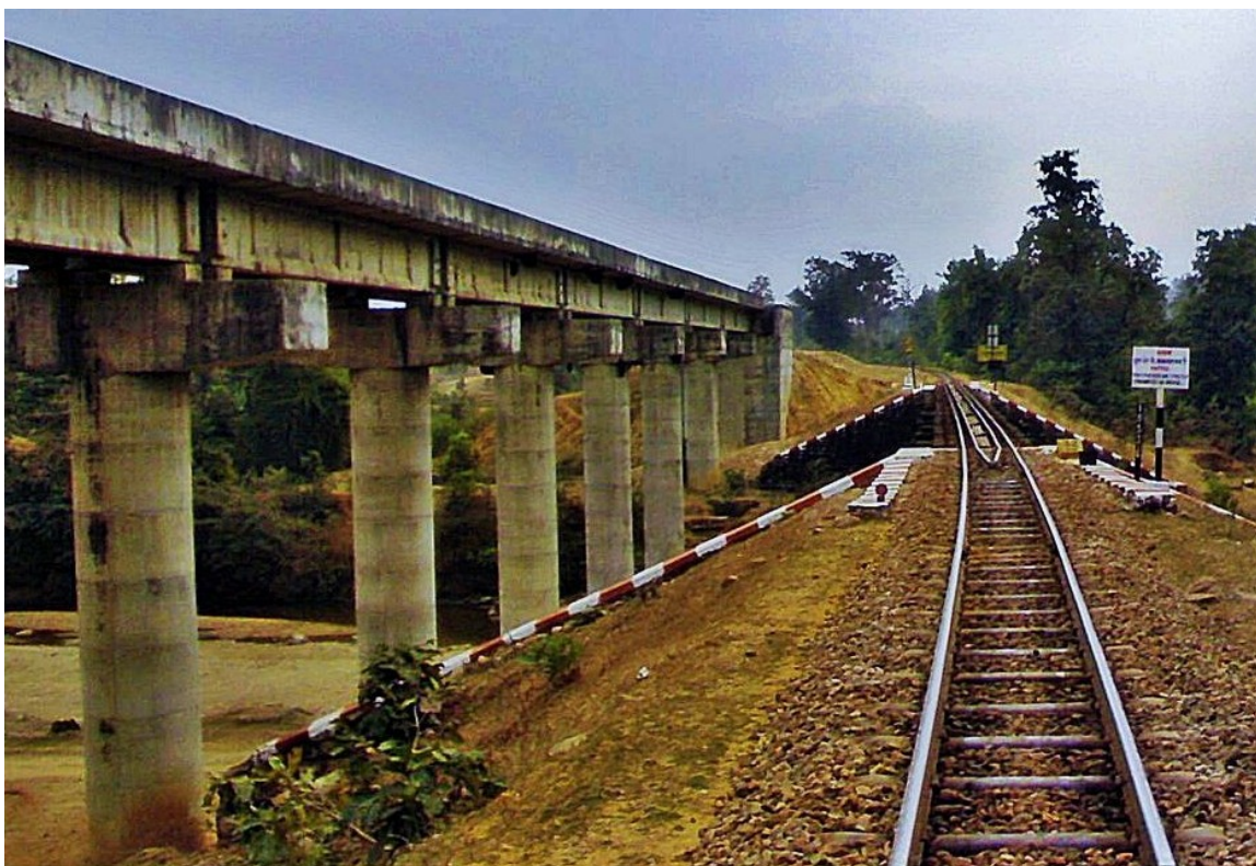
2 ½ ft Narrow to Broad-Gauge Conversion under Progress on the Satpura Narrow-Gauge Network with the focal Point at Nainpur of the once over 1000 km Bengal Nagpur Railway
