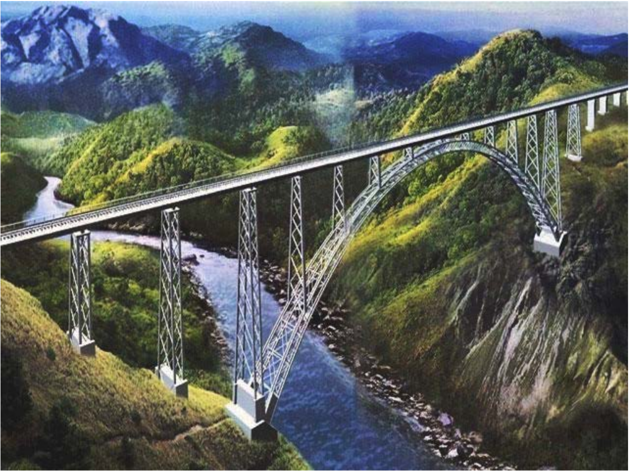
Animation of the Chenab-River Bridge, with 359 m the highest Railway Bridge around the Globe, on the Katra-Banihal Link to Kashmir
