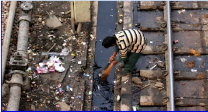
Poorly Drained Track
