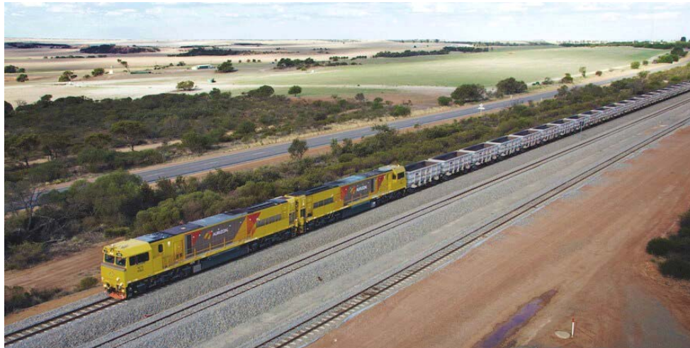
Modern High Quality heavy Haul Rail-Track in Australia
