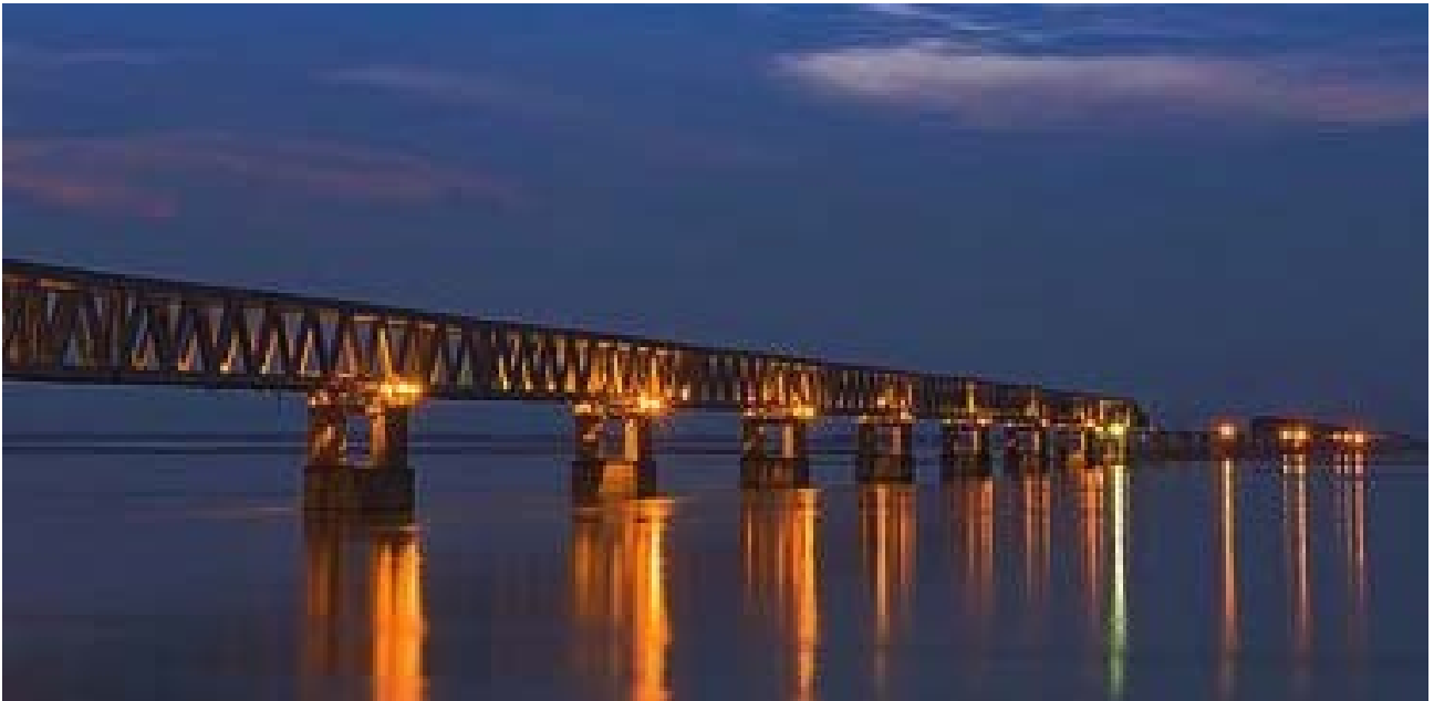
4.94 km long combined Road-Rail Bogibeel Bridge over the Brahmaputra-River under Construction
