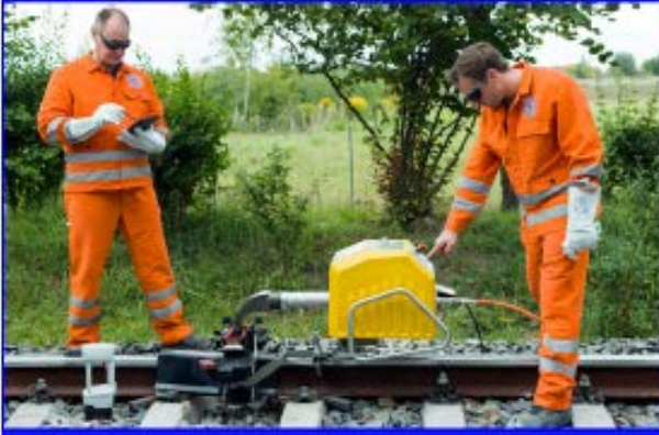
Digital Thermit Welding
