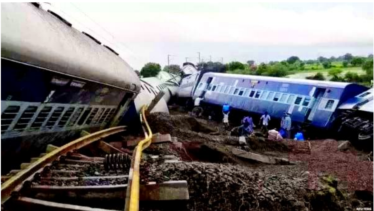
Something went terribly wrong on the Interface of Wheel and Rail on an unhealthy Rail-Track
