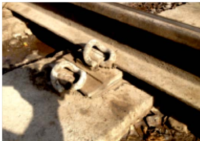
Fig. 7: “Indigenous indirect Fastening System”
