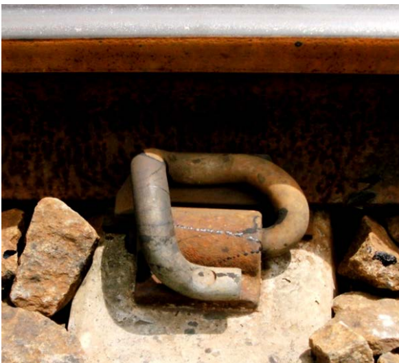
Fig. 2: “Left-handed” MARK III ERC on Indian manufactured IRCON Sleeper
