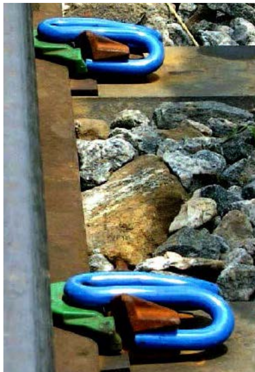
Fig. 6: Fast-Clips on Sri Lanka Railways; Steel-Sleeper and Clips from Pandrol Rahee Technologies Pvt. Ltd.
