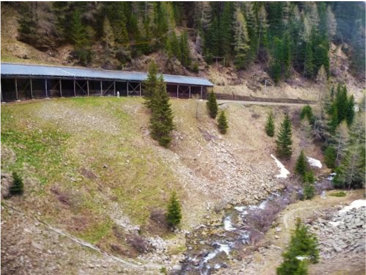
Protection-Gallery, Bernina Railway, Switzerland
