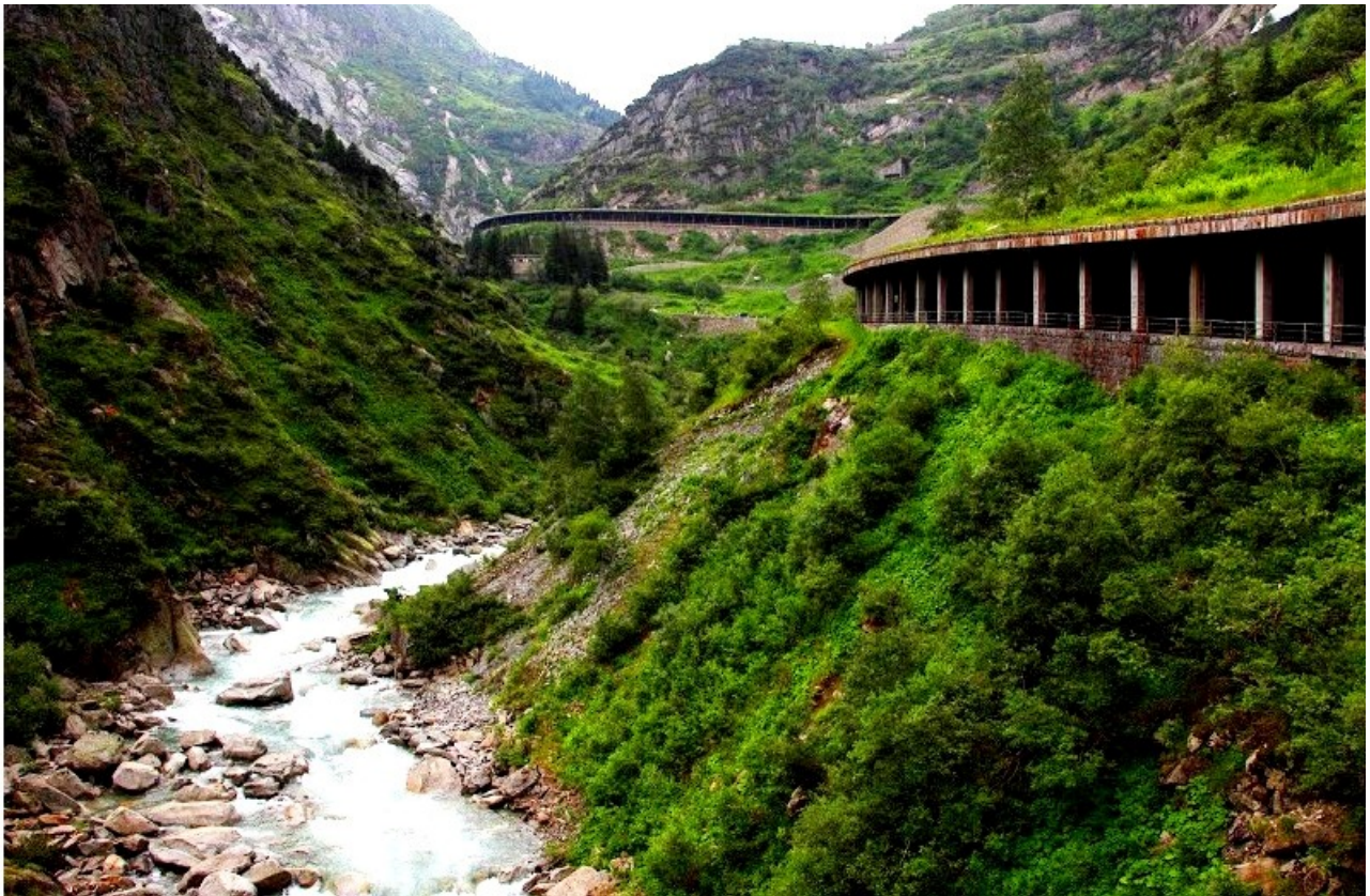
Protection-Gallery; Schöllenen Gorge, Switzerland
