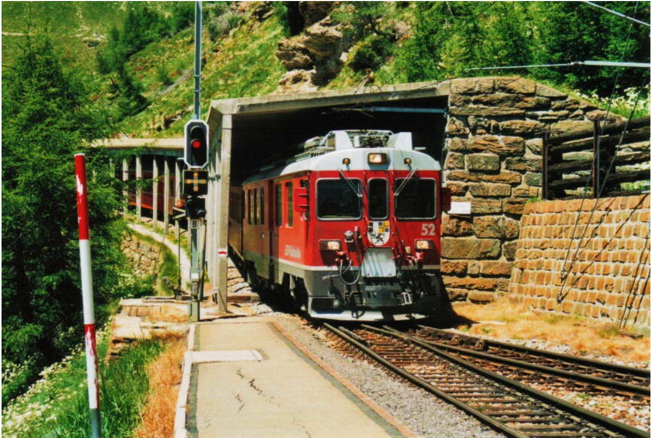
Protection-Gallery, Bernina Railway, Switzerland
