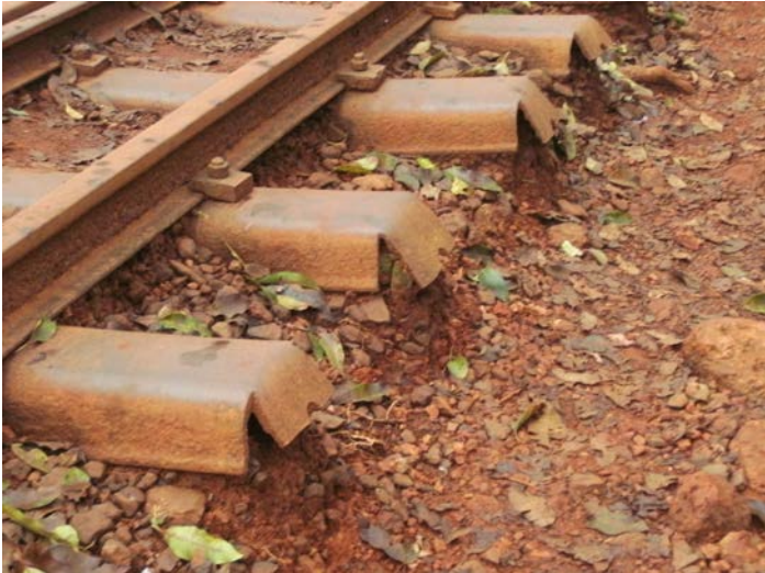
Formation and Ballast missing along the Track
