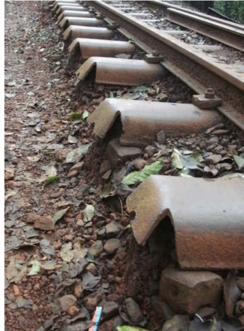
Formation and Ballast missing along the Track
