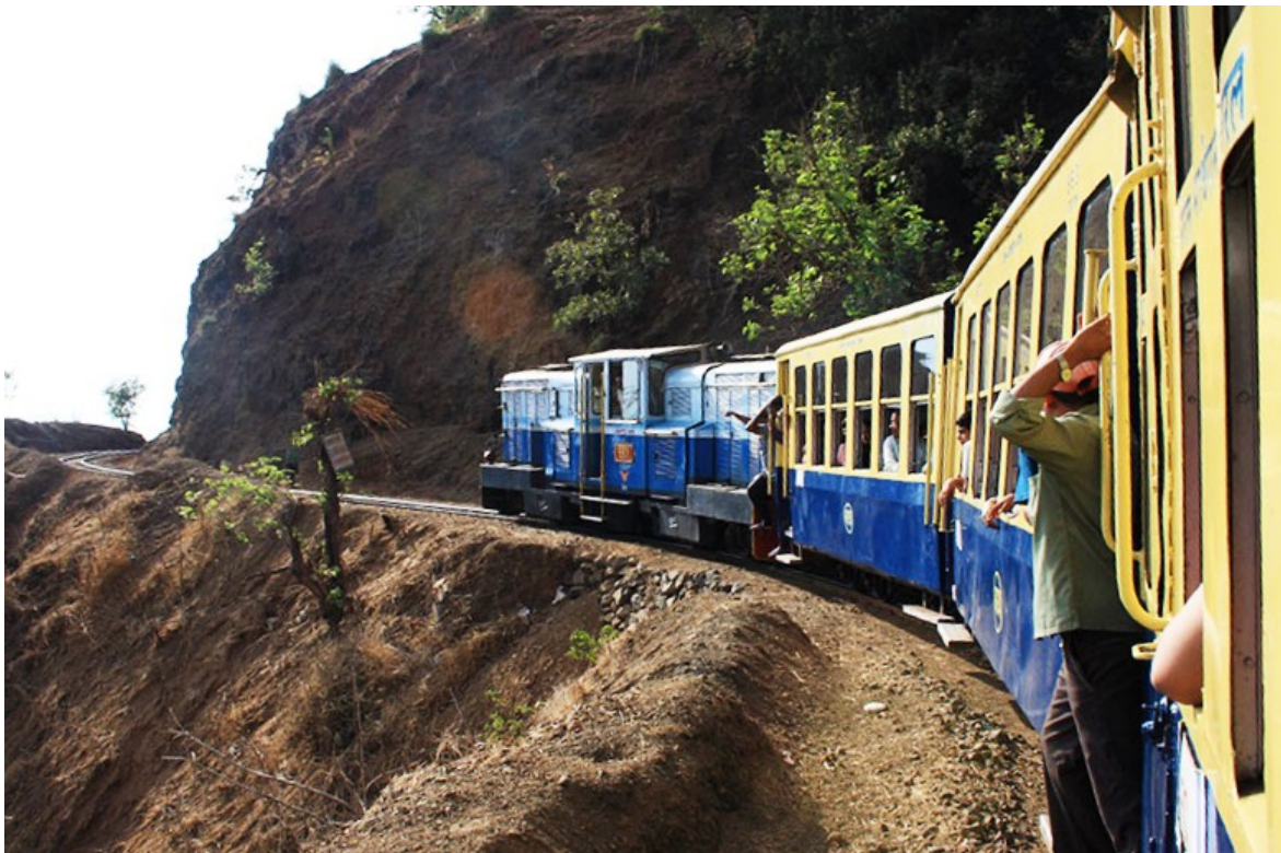
Chuckling around Panorama Point on the Abyss without any Protection Wall and without any Protection Guard-Rail to prevent Derailments and Coaches to tumble down the Precipice
