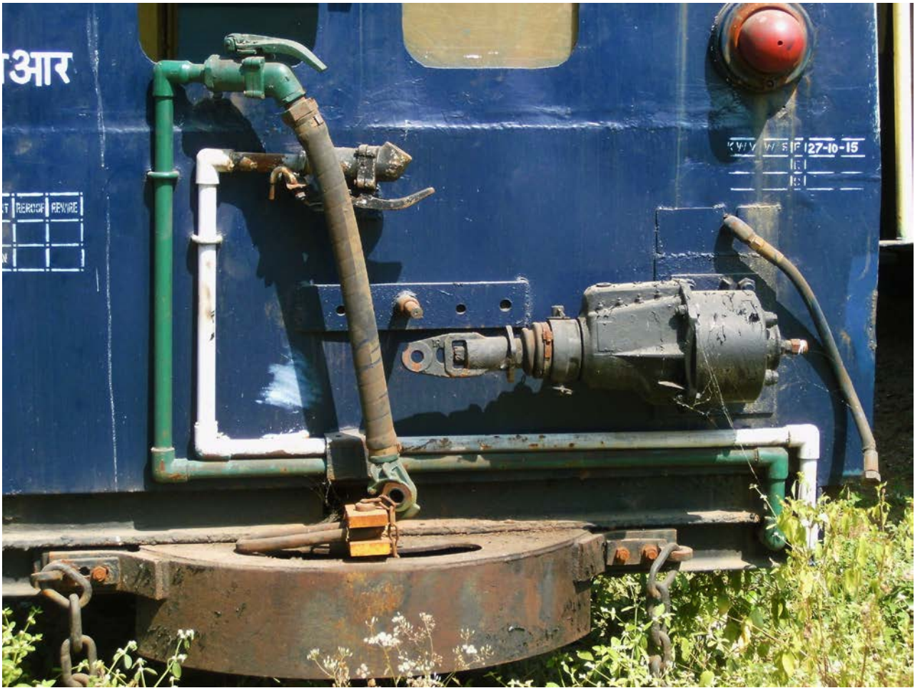
Vandalised Dual-Pipe Compressed Air Brake Components at Neral
